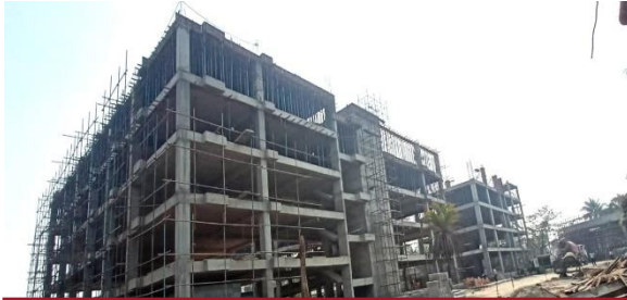
Medical and healthcare facility under construction
